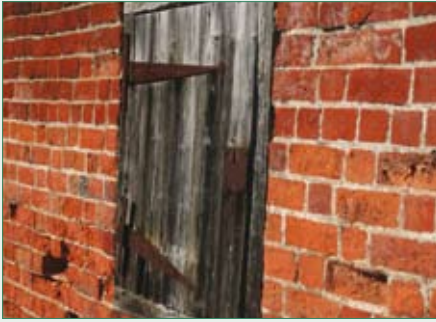
Brick Wall Parkers Lane
